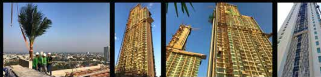
Construction of The Riviera, Wongamat Beach as of February 2017
